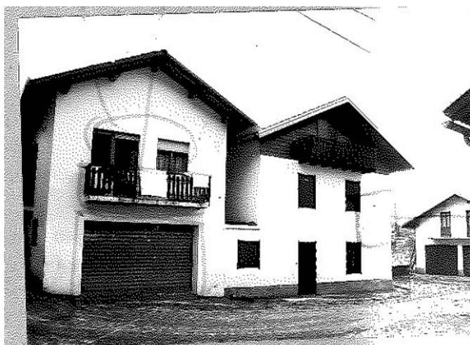
p.ed. 25/1 demolita (Sud) - p.ed. 25/2
